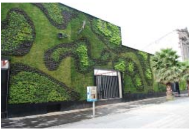
Green wall at the Universidad del Claustro de Sor Juana in the historic center of Mexico City. Source: Wikipedia
